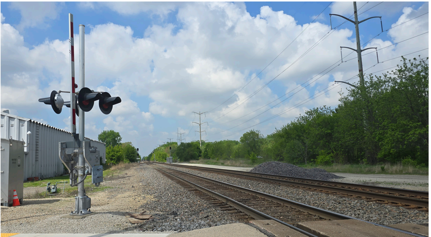
BNSF Railway Crossing
