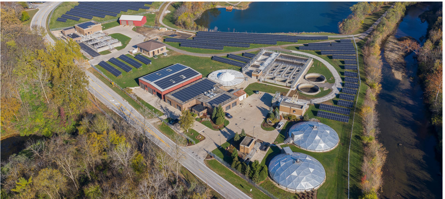
Plano Water Reclamation Facility Image Credit: City of Plano
