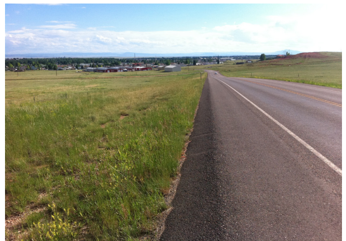
Example of Wider Road Shoulder for Bicycling Image Credit: Alan Levine, Flickr, CC BY 2.0
