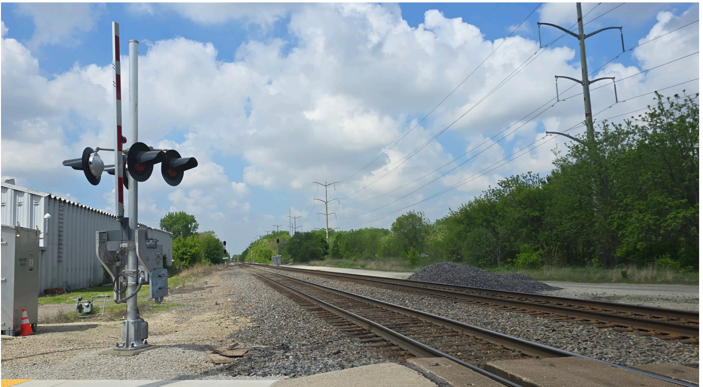
BNSF Railway Crossing
